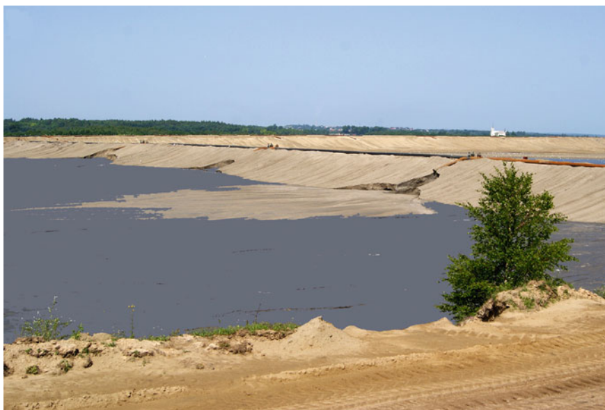
Fig. 8.3 Settling tank after flotation of zinc and lead ores in the Bolesław Mining and Metallurgical Plant (Dulias 2012)
