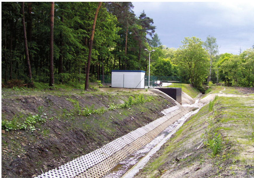
Fig. 5.8 Nowy Dwór watercourse, with paved banks and deepening of the channel to dewater flooded plains in the middle section of the valley (Dulias 2006)
